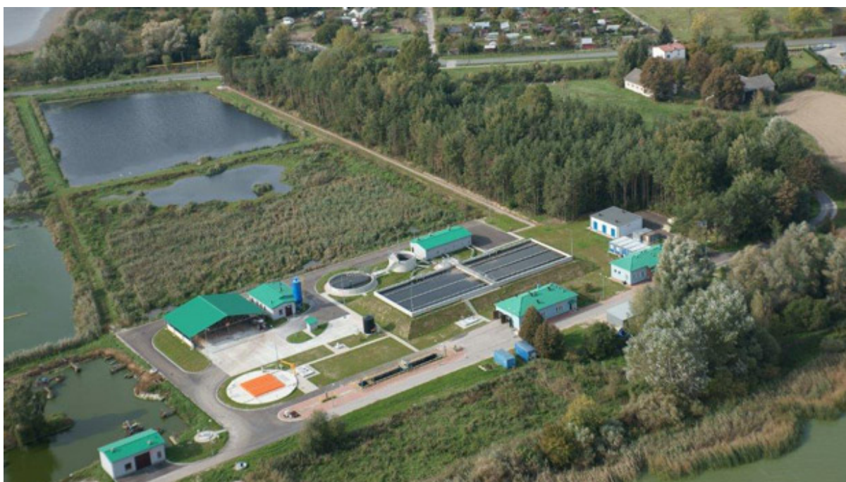
Figure 3: Aerial photograph of Ryki WWTP
