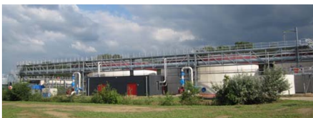
Figure 4: Epe WWTP – First full scale Nereda® Technology Plant
