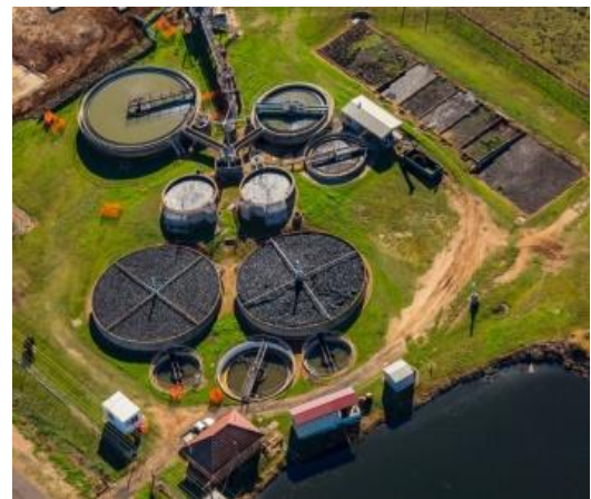
Figure 2: The old Kingaroy WWTP
