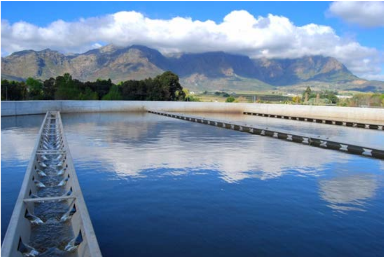
Figure 6: Effluent discharge from a Nereda® reactor at the Wemmershoek WWTW
