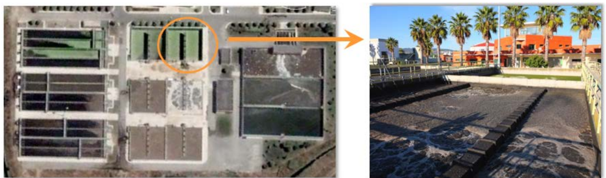
Figure 11. Conversion of reactor n°6 of Frielas WWTP to Nereda ® technology.
