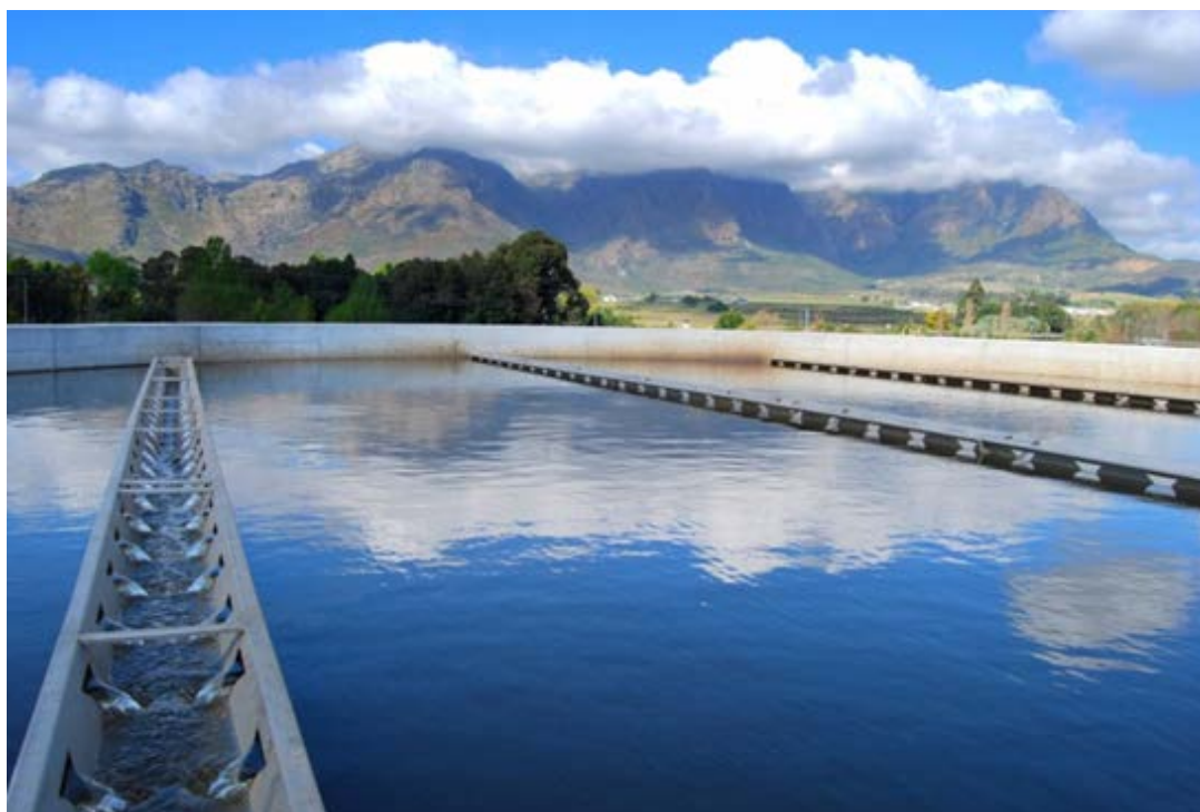
Figure 8. Nereda ® reactor at Wemmershoek discharging effluent.
