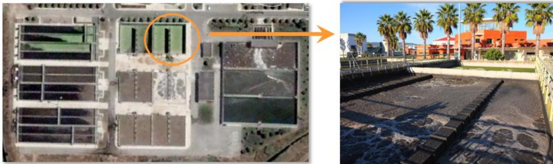
Figure 1: conversion of one of the reactors of Frielas WWTP to Nereda® technology
