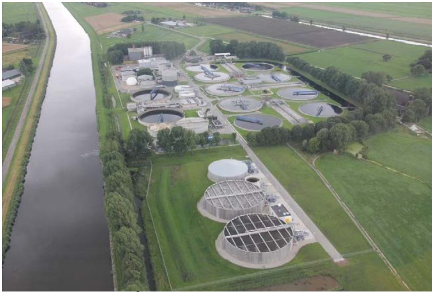
Figure 10 – Nereda ® Garmerwolde WWTP
