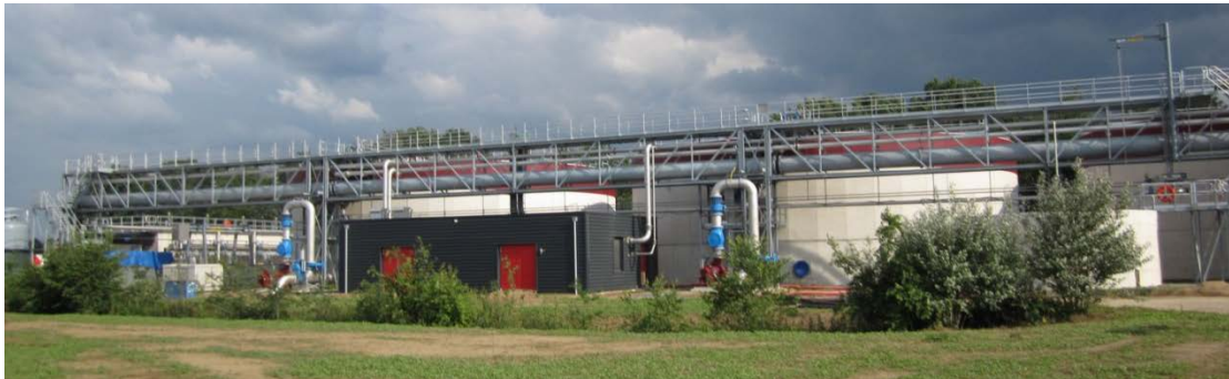
Figure 4: Nereda ® Epe WWTP
