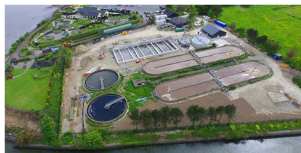
Clonakilty WWTP, with the rectangular Nereda tanks
