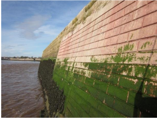
Figure 9 – Reinforced Concrete Repair
