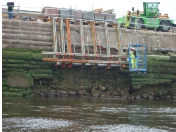
Figure 7 – Manrider Basket Access/ Top shutter Installation
