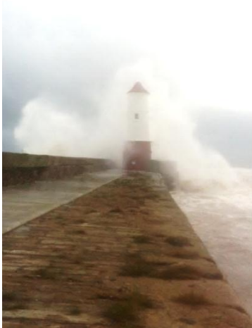
Figure 11 – Breakwater battling the elements
