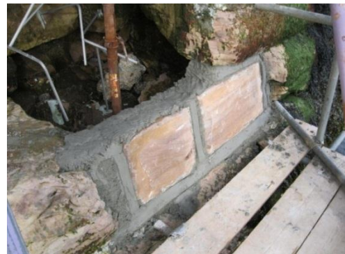
Figure 8 – Blockwork repair mid structure
