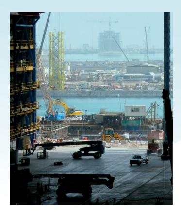
The quays and finger piers enable maintenance work on large ships, and incorporate all required mechanical and electrical services. There are numerous piped systems, distributing all the fluids necessary for ship repair, including acetylene, carbon dioxide, compressed air, LPG and oxygen, in addition to the ballast water and fire fighting systems.
