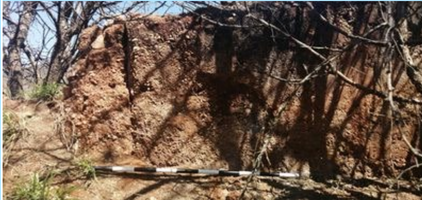
Figure 7-46: Intact walling of the homestead
