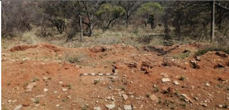
Figure 42 – Poorly preserved historic homestead. Made of mud, stone and cement. Only foundation with bits of crumbled walling have preserved.
