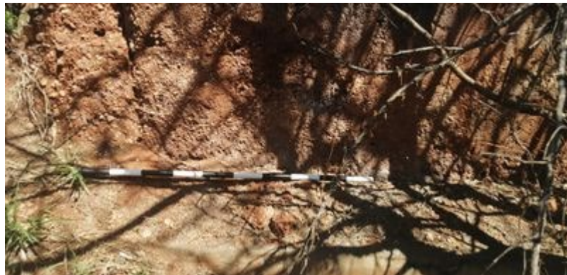
Figure 56 – A view of the intact walling of the homestead.
