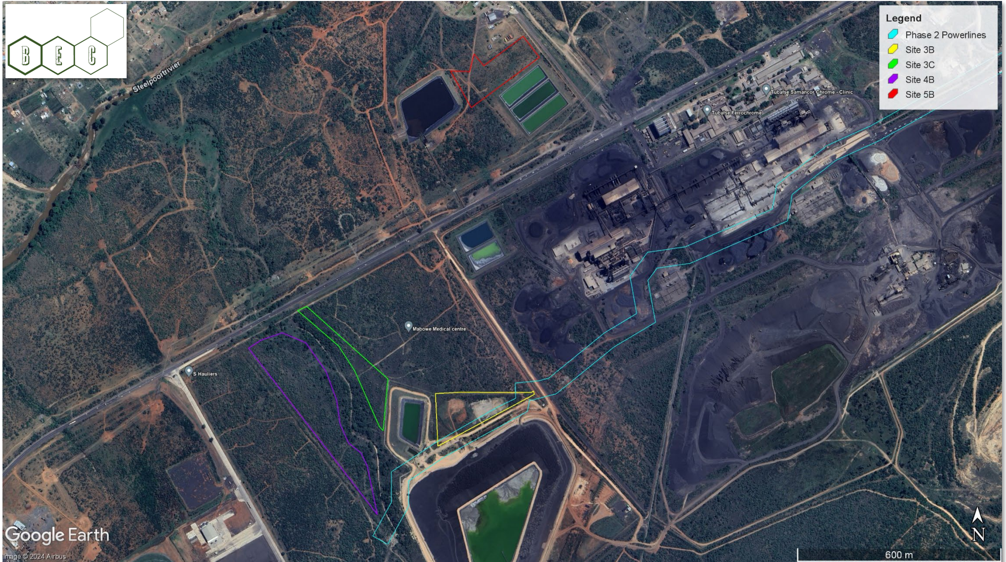
Figure 2: Aerial imagery of the site and immediate surrounds (Sites 3, 4 & 5)
