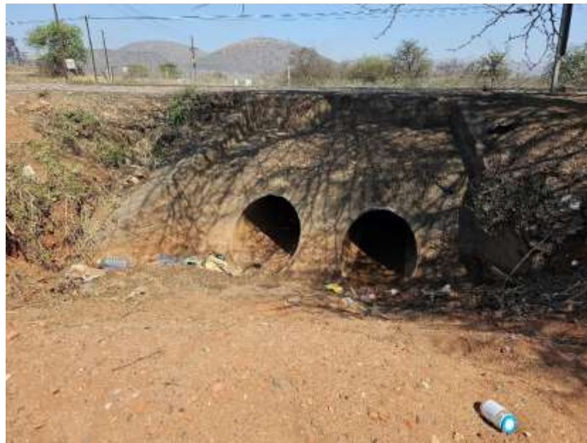
Figure 6-9: R555 double barrel culvert system
